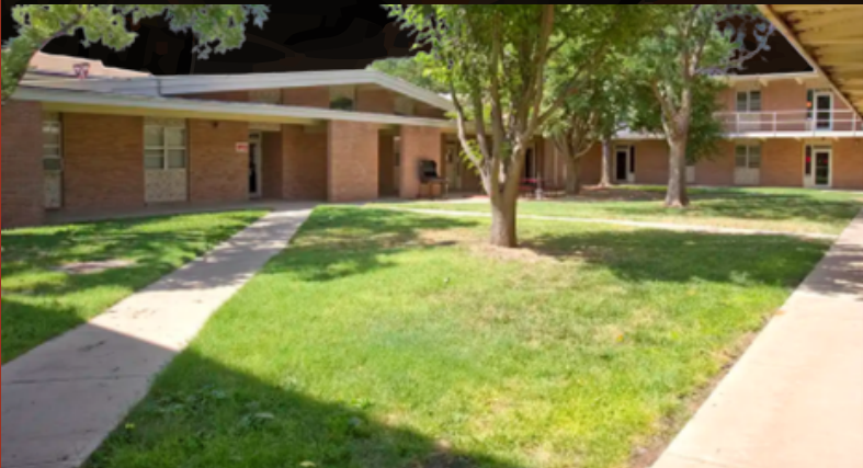
Exterior of Guenther Hall
